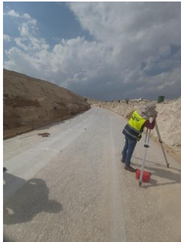
Checking the level of blinding concrete before casting concrete
