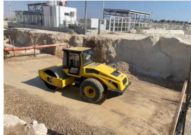
Compaction works under the concrete base for the water channel
