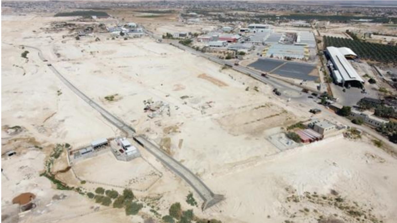
Completed wadi rehabilitation including construction of storm-water channel with a total length of 730 meters
