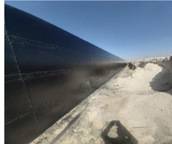
Water proofing works for water channel outside walls
