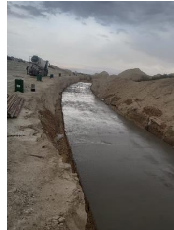
Blinding concrete under the channel foundation
