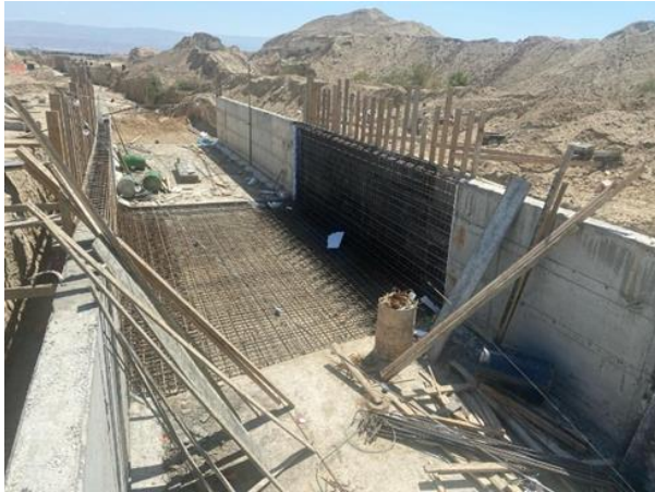
Shutter and steel reinforcement works for the open channel
