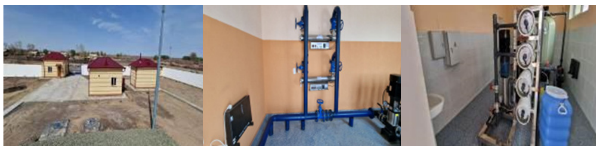
Photos 52, 53, 54: Water project on access to clean drinking water in Taza jol VCC of Chimbay district.
