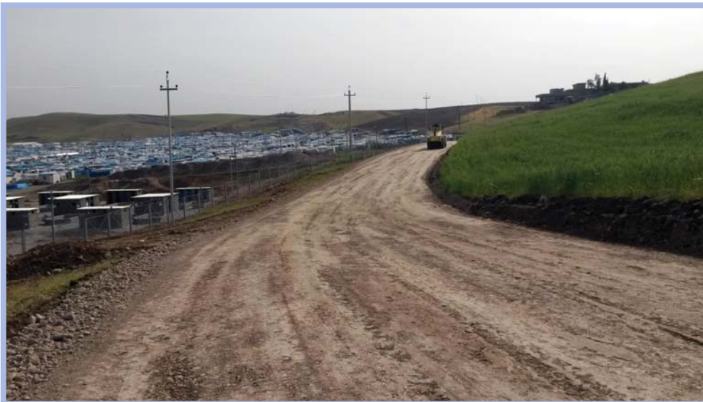
Road constructed in Kawargosk, Erbil.
