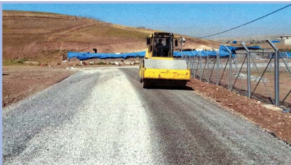
Road constructed in Kawargosk, Erbil.
