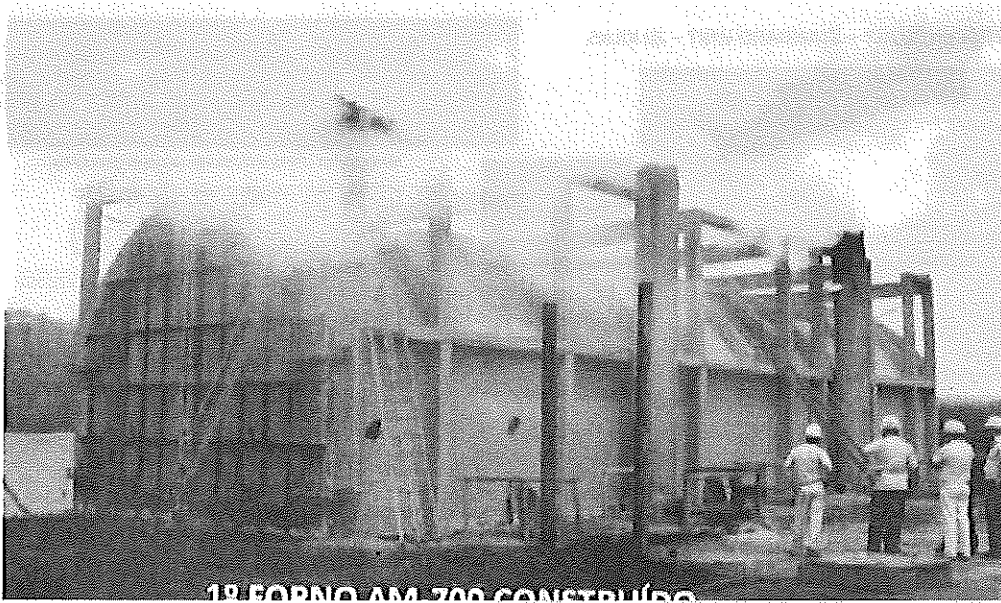
8-5 Big Rectangular brick kiln supported with metal pillars and doors with heat recovery and testing gas capture peripherals.
