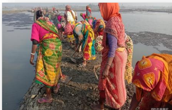
Photo 3: Earthen Road is being constructed under Cash for Work in Shyamnagar Sub-district. District: Satkhira Satkhiara
