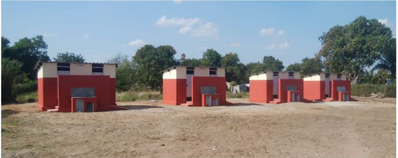
New constructed gender friendly toilets in Chipinde school, Dondo district
