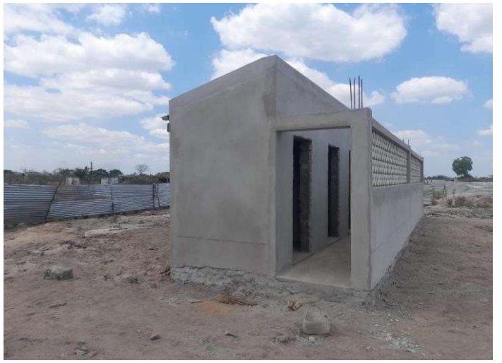
Isometric view of gender friendly toilet at finishing level in Mutua.
