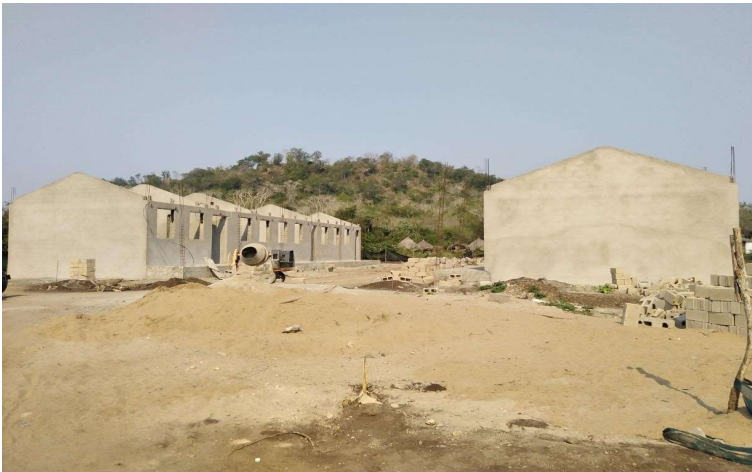
Both school blocks (1&2) are under construction at roof level in Muconja, lot2, Chibabava district.
