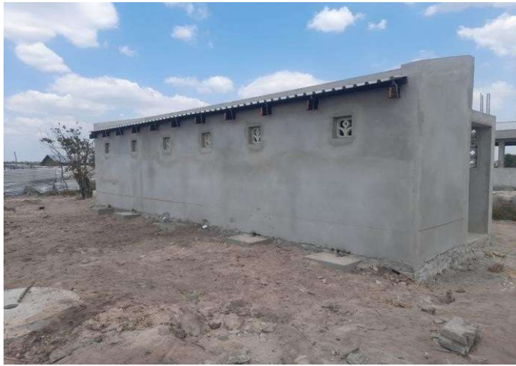
Back side of gender friendly toilet at finishing level in Mutua.
