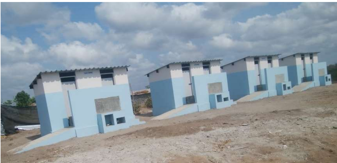
New constructed gender friendly toilets in Mutua school lot4, Dondo district.
