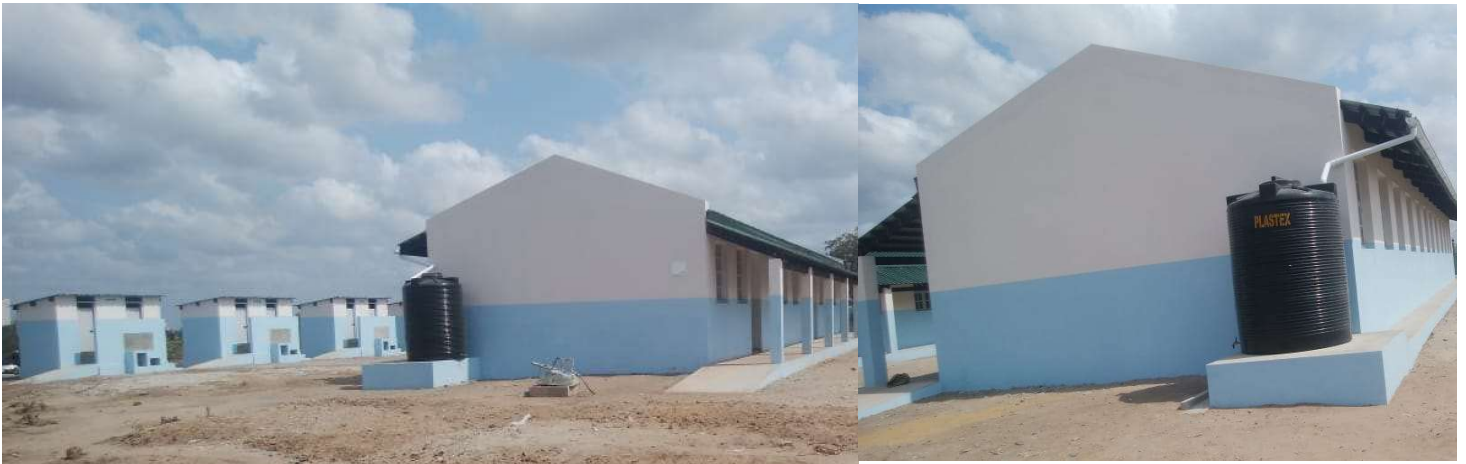
Newly constructed two school blocks in Mutua, lot4 Dondo district.
